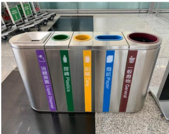
Recycling bins at passenger terminal areas
